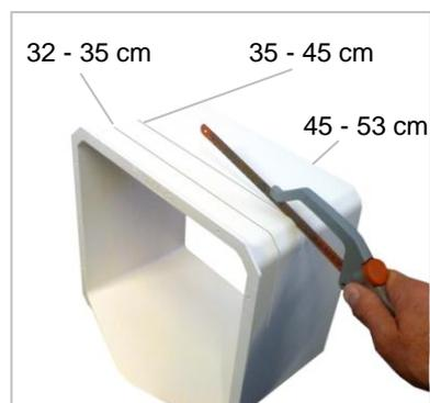
7. The standard separating plate is pre-assembled for wall thicknesses (including stucco) of up to 44 cm.
